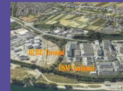
Credit photo DDT68
